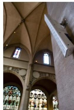
nave loudspeakers with the choir and Lady Chapel speakers on at lower levels; finally, Preset 4 is used for Major events, with all loudspeakers optimised to provide full coverage.
