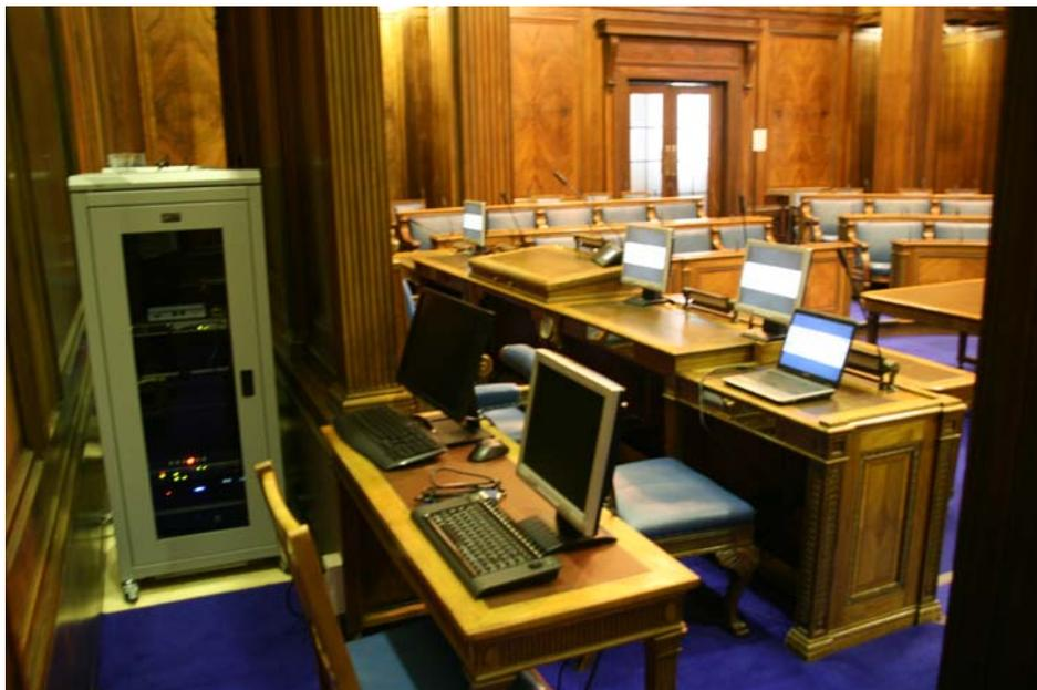
The main equipment rack is hidden behind the screen at the top table and in the foreground is the operators table with full touch screen control of the chip card registration and microphone management. The other monitors relay the video showing on the projectors to the chairman and top table delegates.
