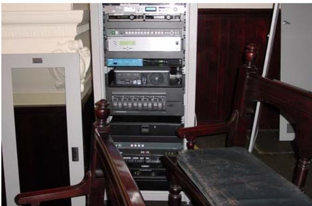
There is no room at the delegates positions to locate individual loudspeakers so a BI amp Nexia CS provides the digital processing and audio control. QSC amplifiers provide the power to 4 Bosch line array columns.
