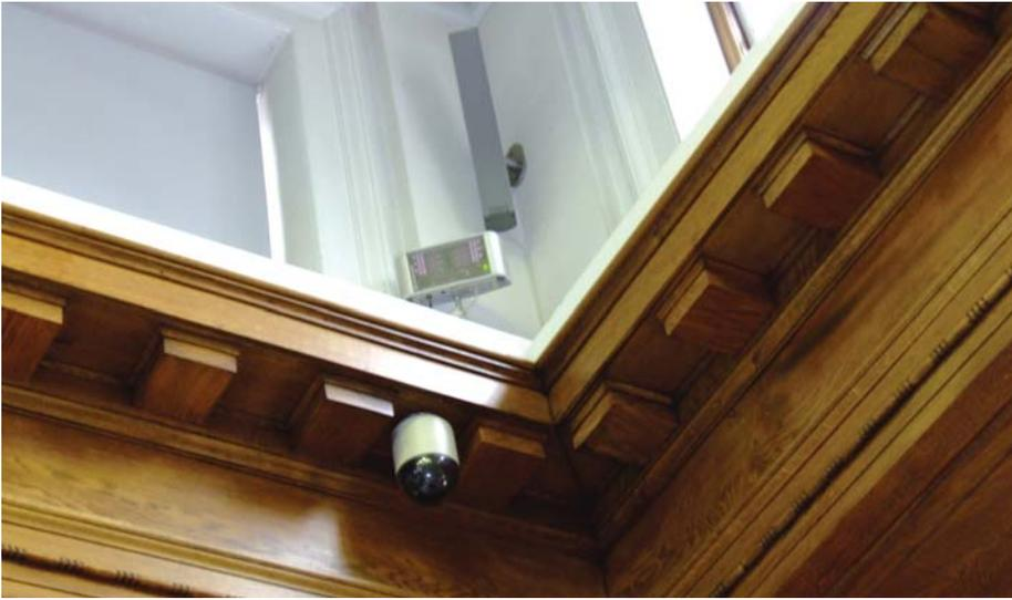
The dome cameras, IR emitters and column speakers are positioned high in the ceiling largely out of sight but still providing good coverage.
